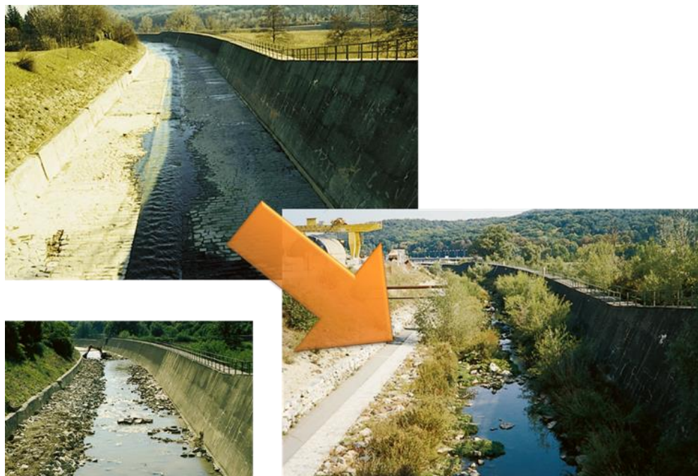
Figure 18. Example of a bioengineering measure for river engineering, demonstrating the transformation from a heavily channelized, concrete-lined river to a restored, vegetated watercourse with improved ecological function.
