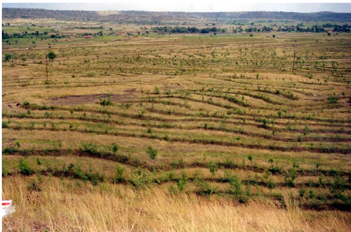
Figure 9. Early-stage construction of continuous contour trenches and plantations.
